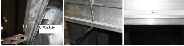
7. Insert the white nylon track insert in the lower track flush to the track ends and temporally hold with vice grip.
