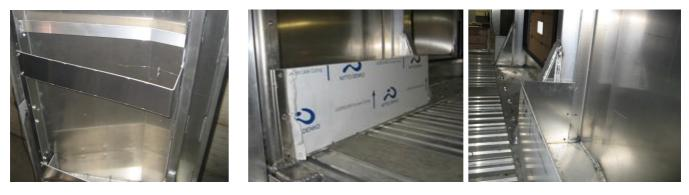
3. Attach the track guard holder to the head board at 20 inches from the base plate
