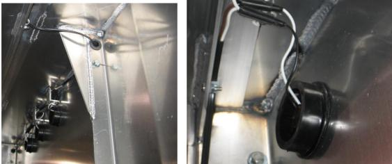
Feed the end of the harness through the hole in the corner of the headboard
